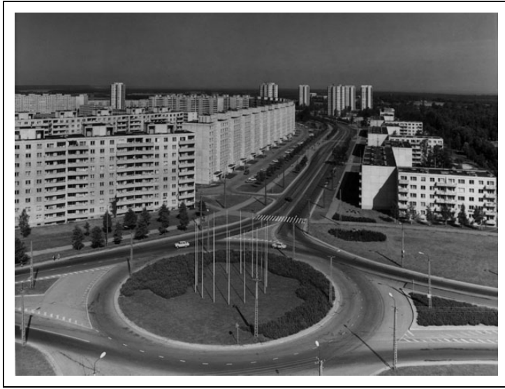
Figure 4. Broad Streets serve residential buildings in Väike-Õismäe, Tallinn, Estonia. An encircling ring road is designed to accommodate motor vehicle travel, preserving the makrorayon interior for pedestrian movement. Photograph by Johannes Külmet.
